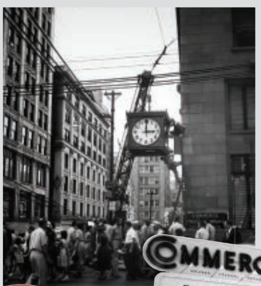
1953 Commerce installs landmark clock at corner of 10th and Walnut. With a weight of approximately two tons, many terrified pedestrians refuse to walk under it.
